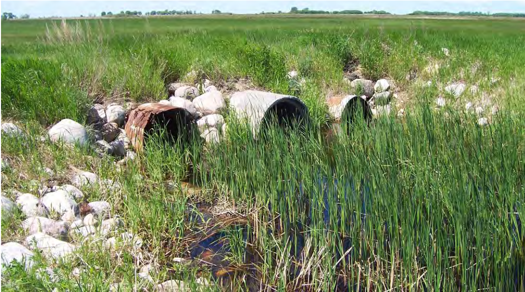
Photo 3.9 – Drain and Culvert near Lake Manitoba
