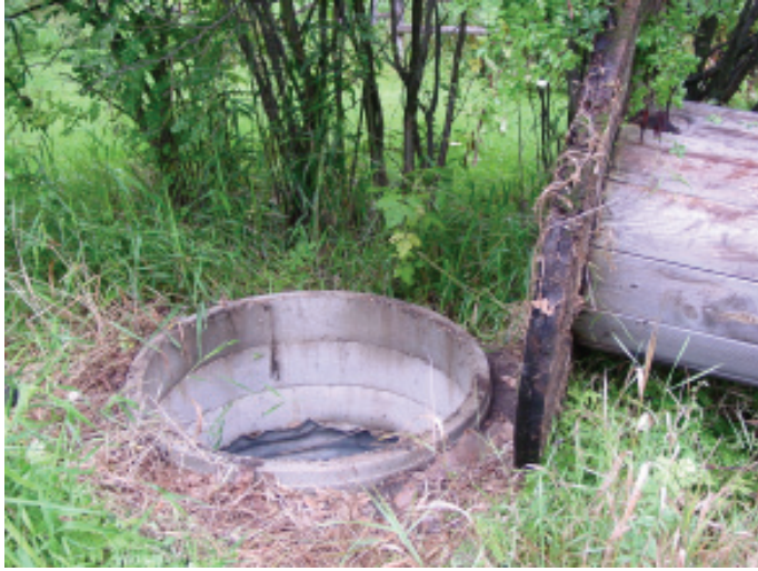
Abandoned wells can act as direct conduits for contaminants from the surface into aquifers.
