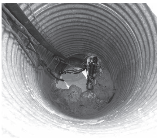
Drilled well in a pit.
