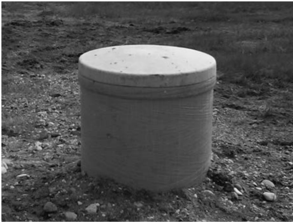
Above: Vermin-proof cap for dug or bored wells. Credit: Manitoba Water Well Association Below: Vermin-proof cap for drilled wells.
