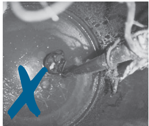
Surface water in well pit.
