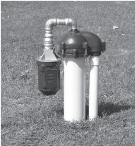
Drilled well with flood-protected cap
