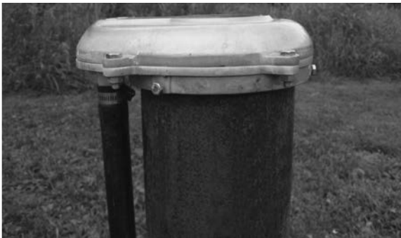
Above: Vermin-proof cap for dug or bored wells. Credit: Manitoba Water Well Association Below: Vermin-proof cap for drilled wells.
