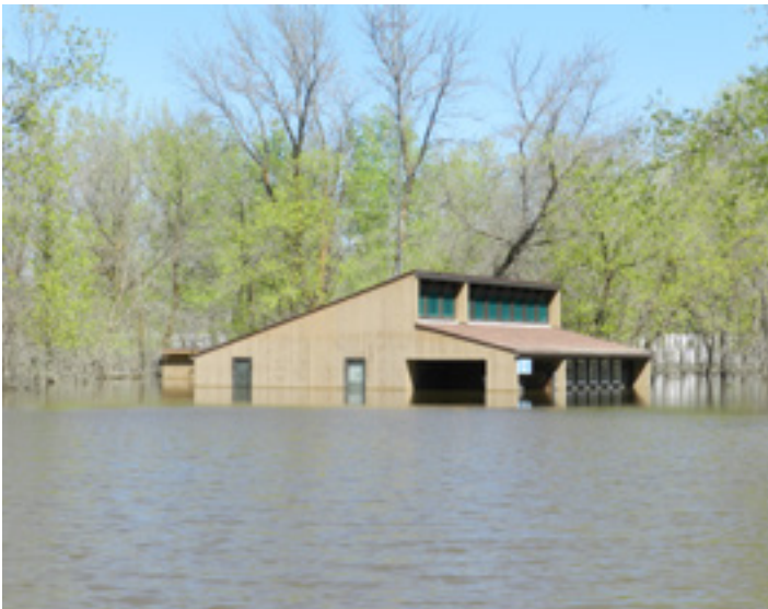
Flooded campground office - 2011
