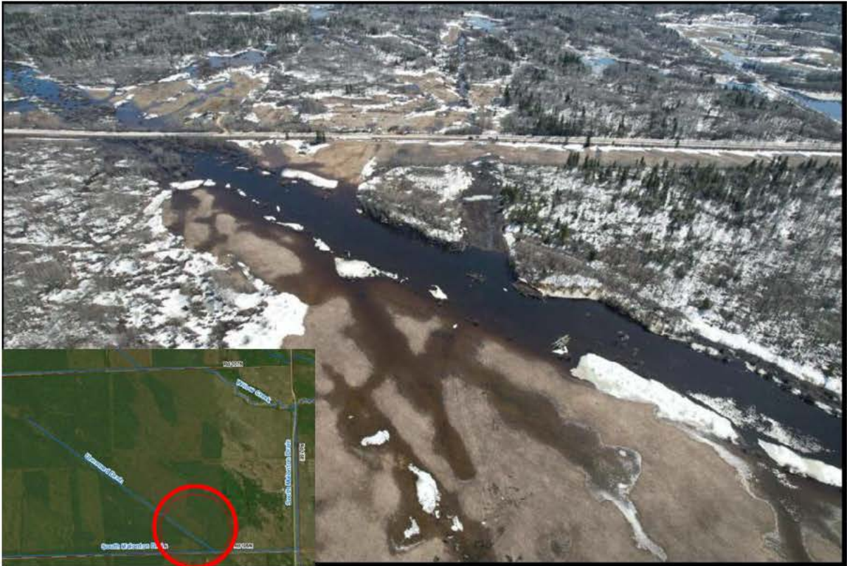
Photo No. 3: Unnamed Drain at Existing Access Road (looking south toward Rd 106N) – Spring 2022 (Photo provided by BMCL)
