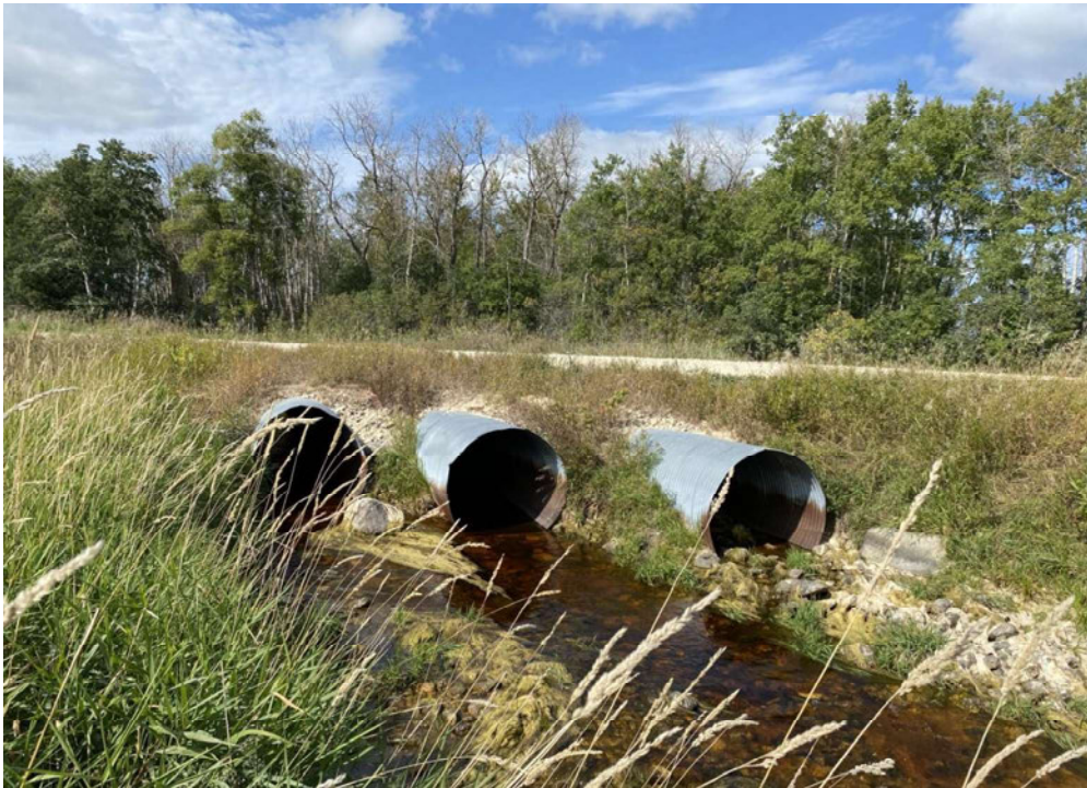
Photo No. 8: Willow Creek South of Rd 107 N (looking upstream) – September 13, 2022
