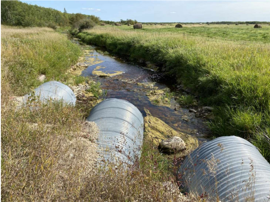
Photo No. 8: Willow Creek South of Rd 107 N (looking downstream) – September 13, 2022
