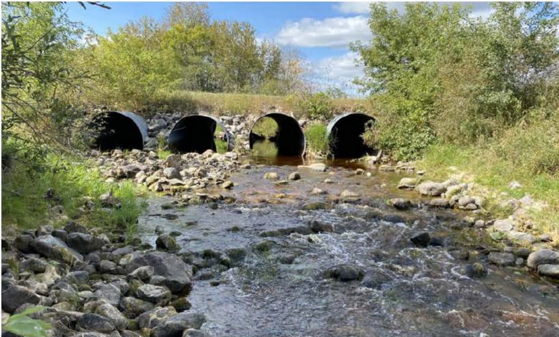
Photo No. 6: Willow Creek East of Rd 15E (looking upstream) – September 13, 2022
