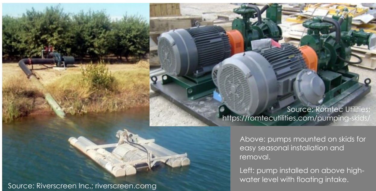
Figure 2.3 Examples of typical pump installations
