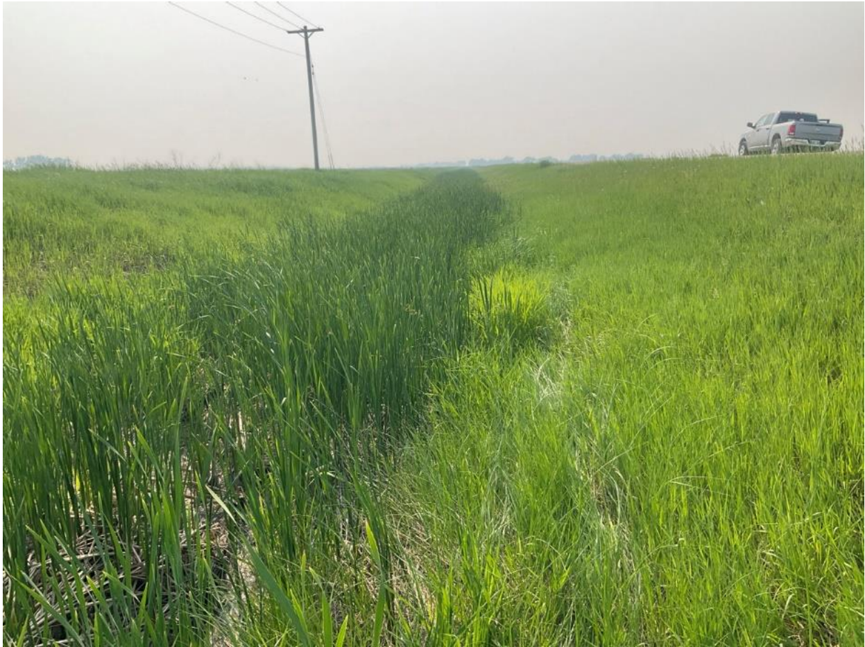
Photograph C-20. Looking west at the east end of WC-29. The channel was vegetated with cattails with shallow standing water and no observed flow at the time of assessment June 5, 2025).
