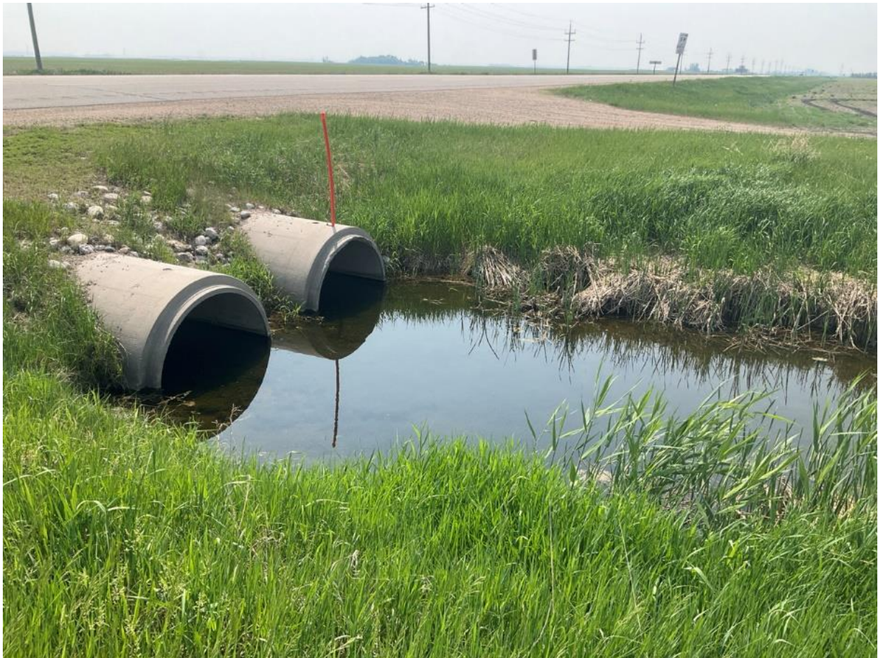
Photograph C-12. Looking SE at the east end of WC-24. Most of the roadside channel was vegetated with cattails and contained shallow standing water at the time of assessment (June 4, 2025).
