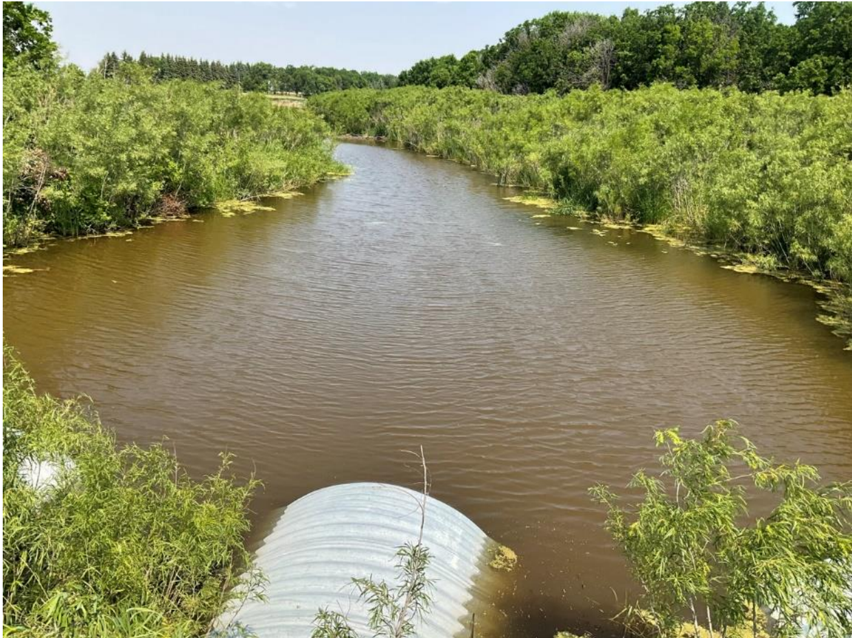
Photograph C-21. Looking downstream at the crossing at St. Adolphe Coulee (WC-31) June 5, 2025).
