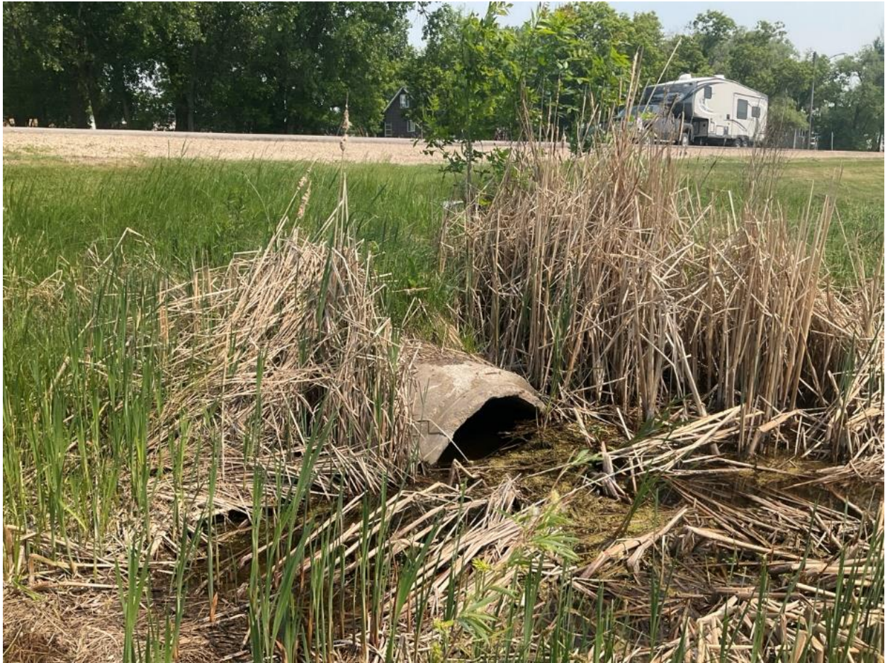
Photograph C-16. Looking northeast at WC-27 on the south side of the road. The channel was vegetated with cattails and contained deep standing water at the time of assessment. No flow observed (June 5, 2025).
