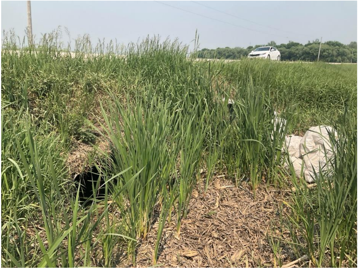
Photograph C-18. Looking northeast at WC-28 on the south side of the road. The channel was vegetated with cattails and dry at the time of assessment (June 5, 2025).
