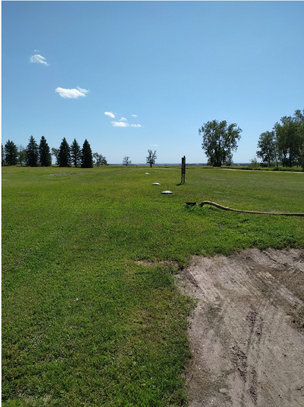
Photo C - Receiving Pipe, 4500 Liter Tank, 3500/1000 Liter Tank, Switching MH, Mound in Distance
