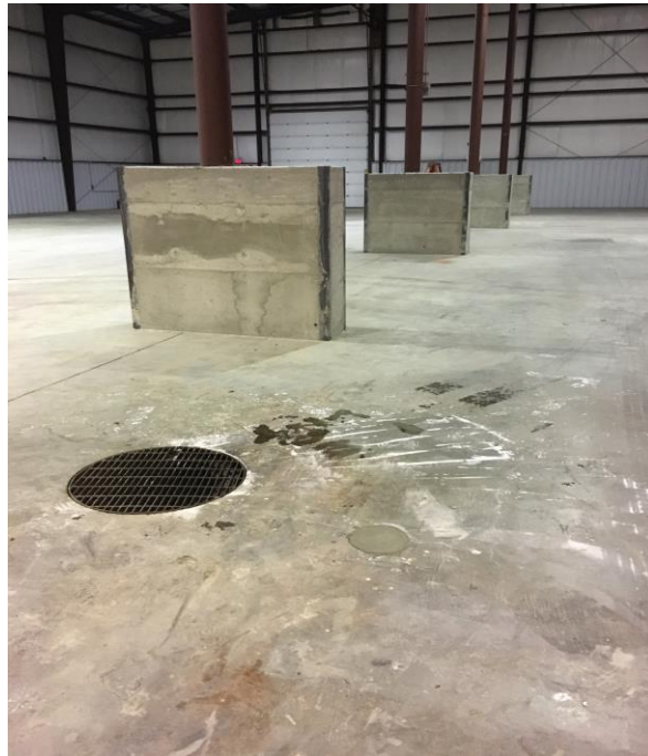
Photograph 1: Monitoring well TH19-11 inside building on site.
