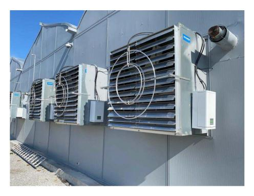
Photo 1 – Example Installation of Bektra RV5 Fans LP PR2182M System.
