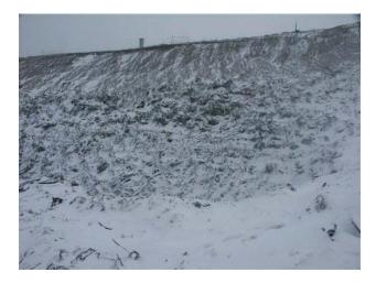
Figure 2. Slope steepened to 1H:1V
