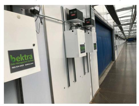
Photo 2 – Example Installation of Bektra LR Corridor RV5 Roof Mount Fans System.
