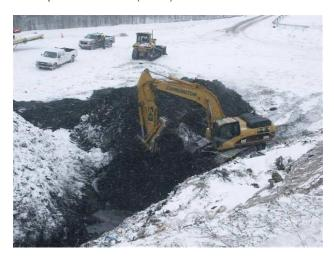
Figure 1. Excavation in progress at the south slope of Barrie landfill.
