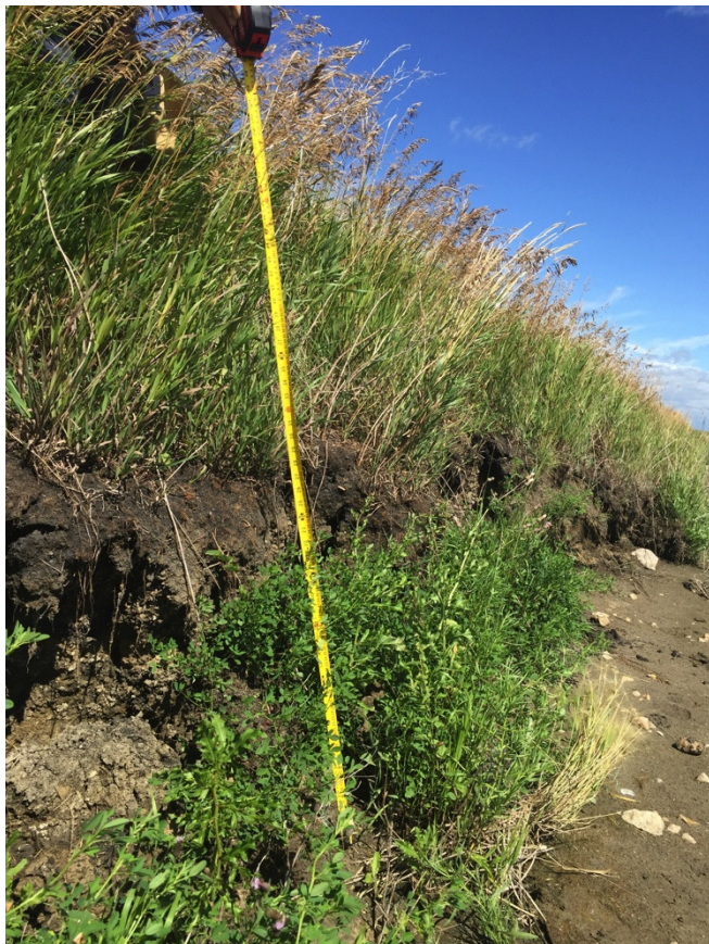
Figure 1 Erosion Secondary Cell
