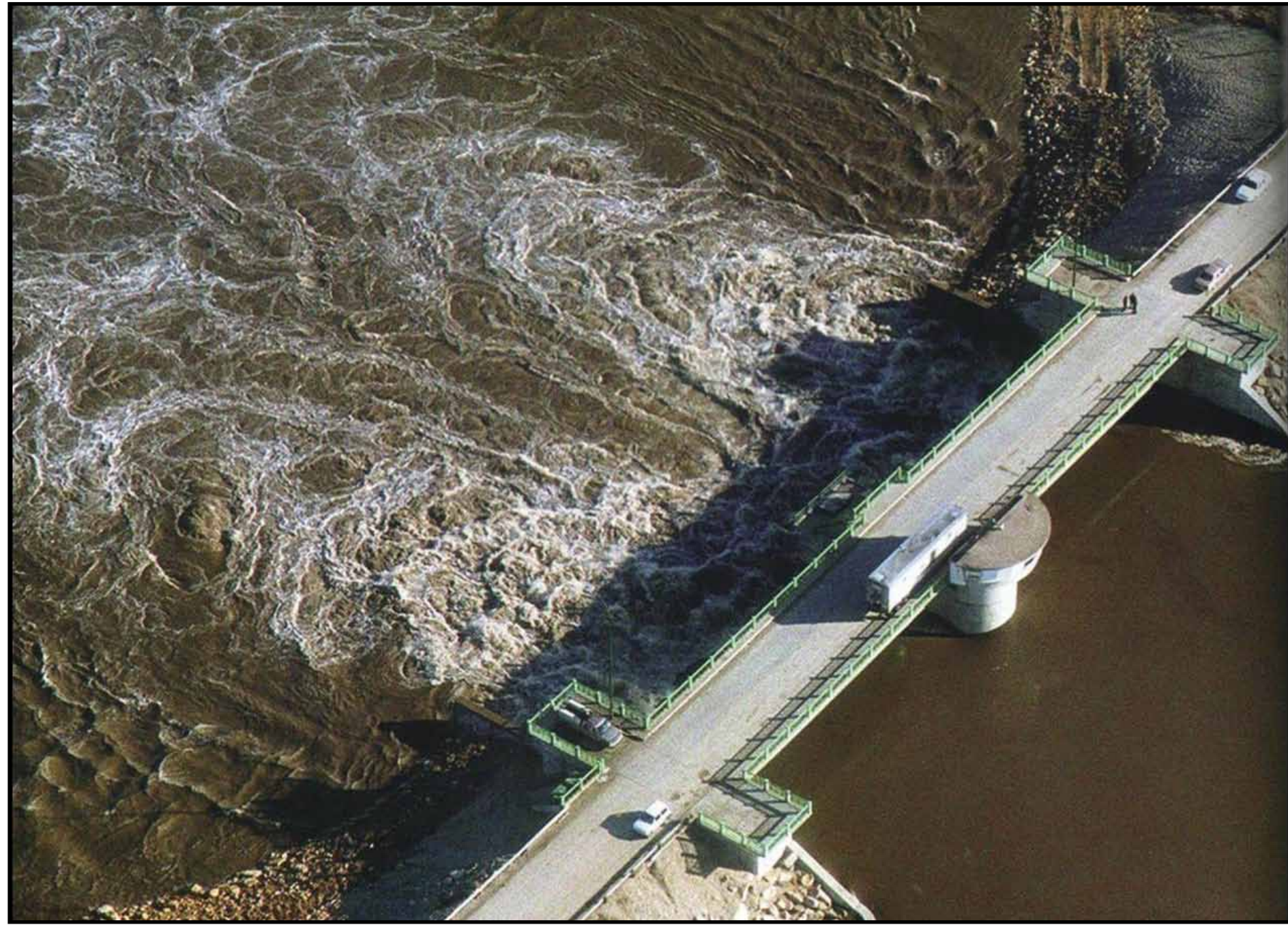
Floodway inlet control structure
