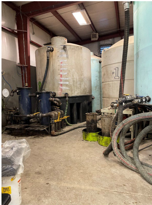
Photo 3 – View of additional pre-existing tanks in Building B at the Facility.
