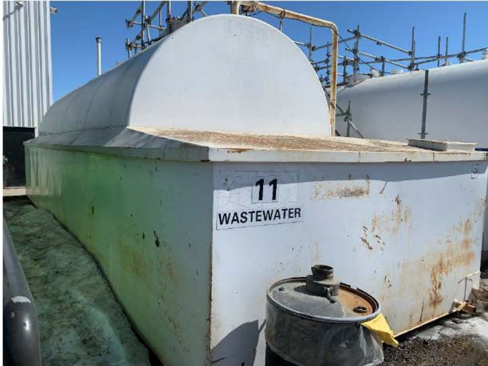
Photo 1 - 50,000 L AST that will be brought to Site.
