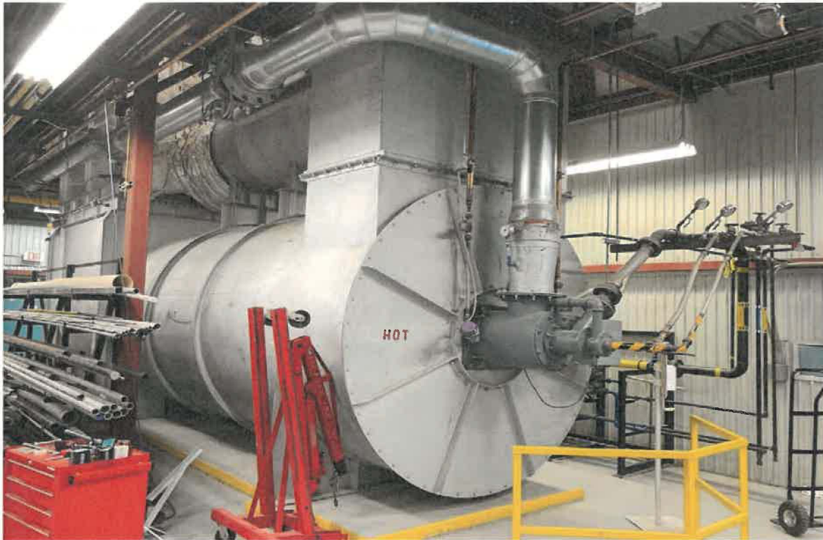
Figure 2–1 Existing Thermal Oxidizer
