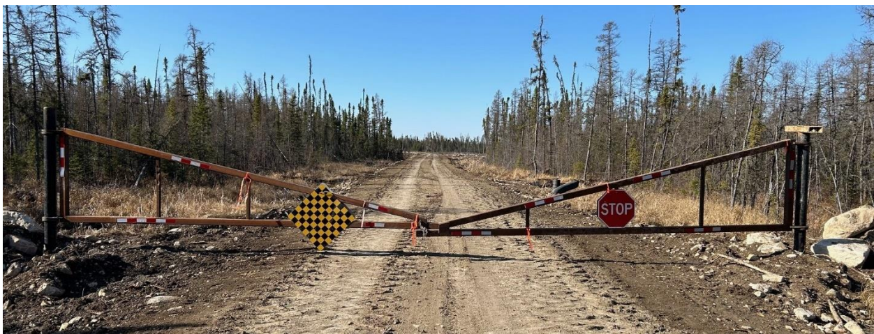
501 502 An example of locked road gate that may be used to restrict access to a Canadian Kraft Paper Industries Ltd road.
