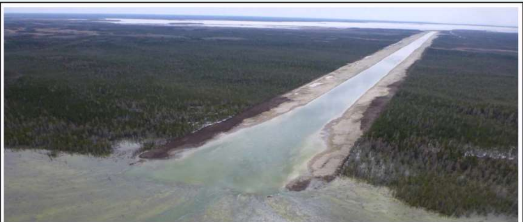
Lake St. Martin Emergency Outlet Channel ( Fall 2011 )
