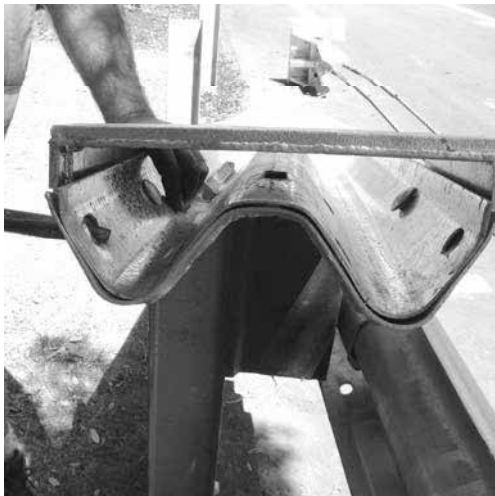
Figure 12. Sit rail 1 so it is raised off the ground.
