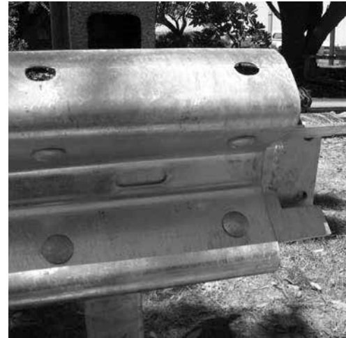
Figure 11. Remove angle bar bolts.
