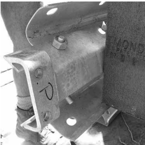
Figure 10. Bolt Slider Bracket to end of rail 2 at post 3.
