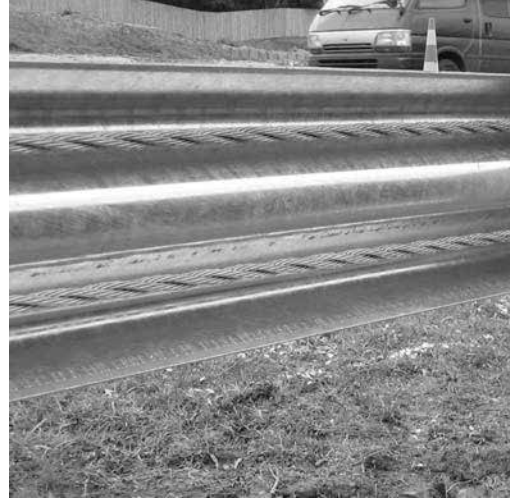
Figure 26. Tighten cables until they are taut.
