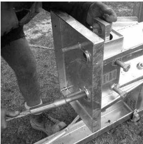
Figure 21. Pass the cable through the bottom hole.
