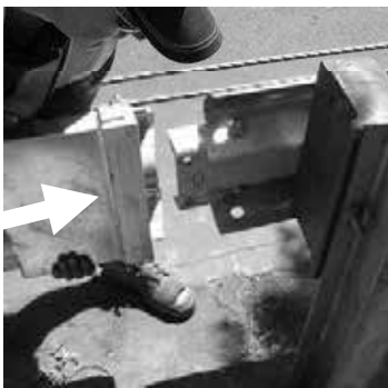
Figure 14. Push Slider Panel over rail 2.
