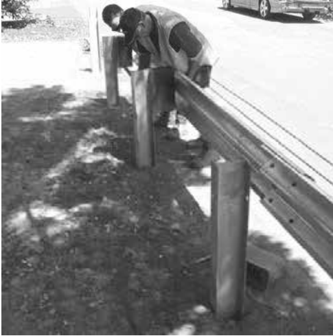
Figure 8. Bolt rail 2 to post and blockouts.
