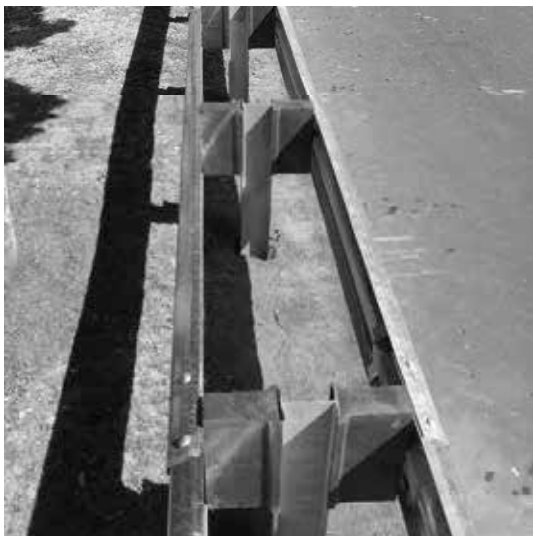
Figure 37. Rails installed with blockouts.
