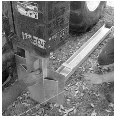
Figure 5. Drive post 1 into augured hole.
