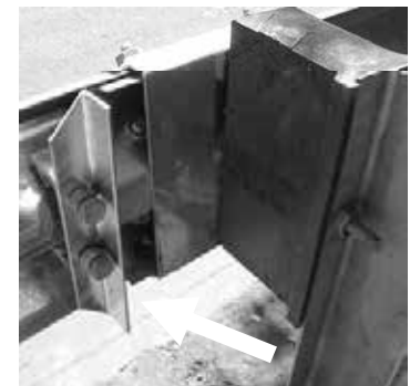
Figure 16. Reattach the angle bar.
