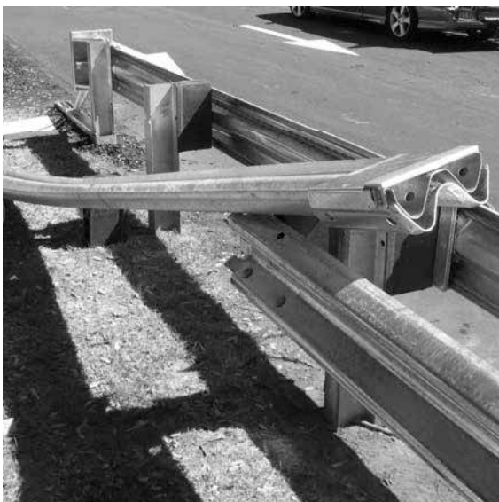
Figure 41. Fit the Slider Panel onto the straight end of rail.
