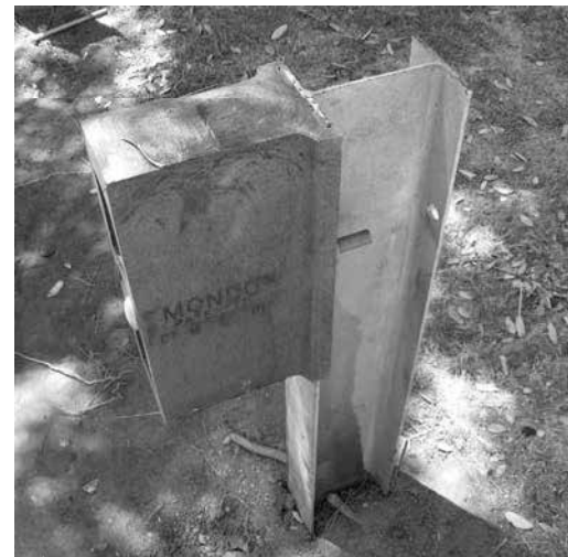
Figure 3. Bolt the blackout to post 3 prior to attaching the rail.
