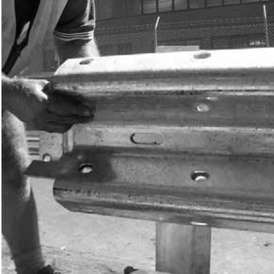
Figure 39. Bolt Slider Bracket to upstream end of rail 2.
