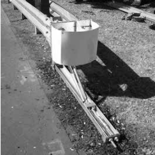
Figure 47. Attach nosing using nylon push rivets.
