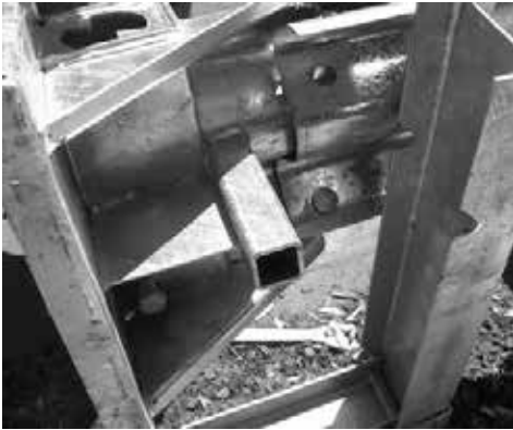
Figure 17. Attach Impact Head to rail 1.
