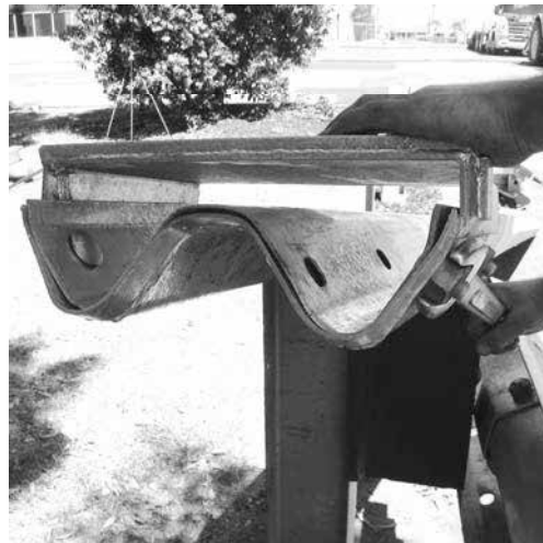
Figure 13. Slide the Slider Panel onto downstream end.
