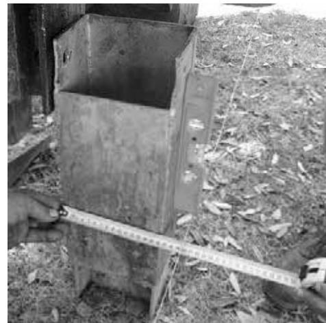
Figure 30. Place roadside face of post 1 towards roadway.
