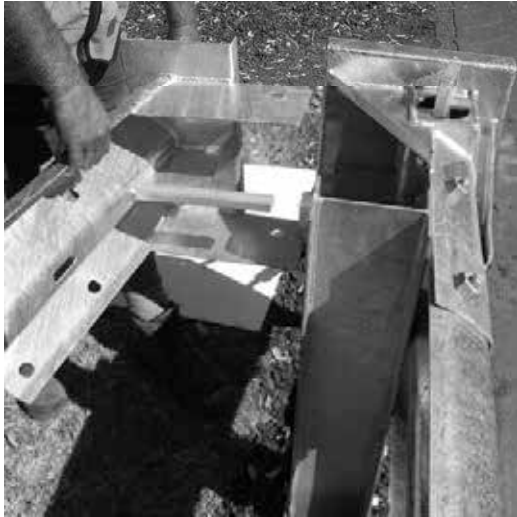
Figure 35. Fit secondary head to main head.
