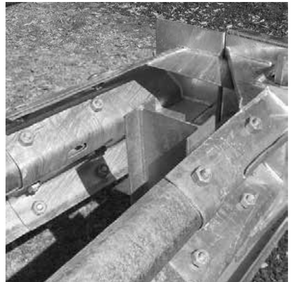
Figure 46. Use 8 standard splice bolts.
