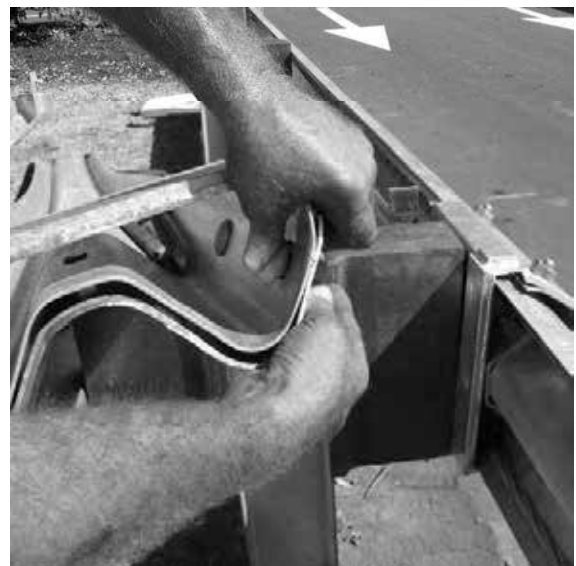
Figure 42. Push bolt from inside (nut on traffic face).
