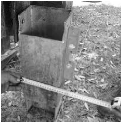
Figure 4. Measure 8 in. towards roadway.
