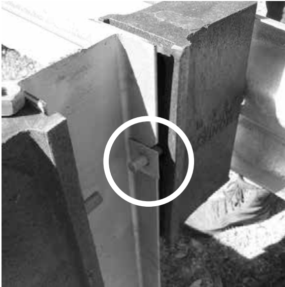
Figure 43. Bolt rail 1 and blockout to post 2 using the square washer.
