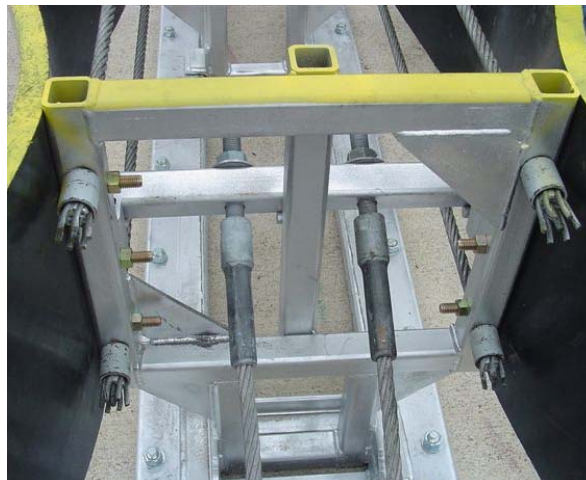
Figure 14 – CABLE INSTALLED IN FERRULE
