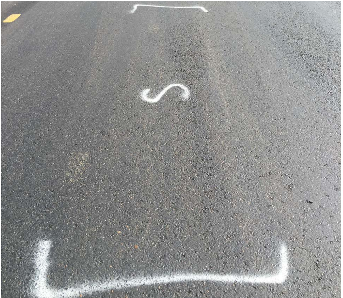
Figure 2 - Slight Segregation
