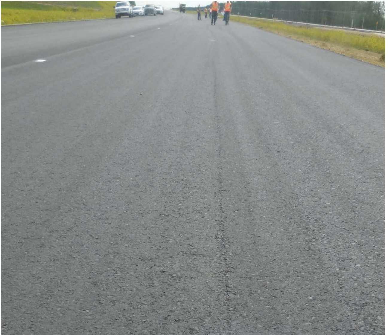
Figure 13 - Paver Streak
