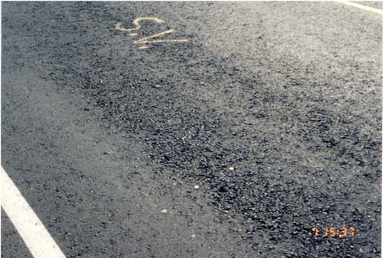
Figure 11 - Severe Segregation
