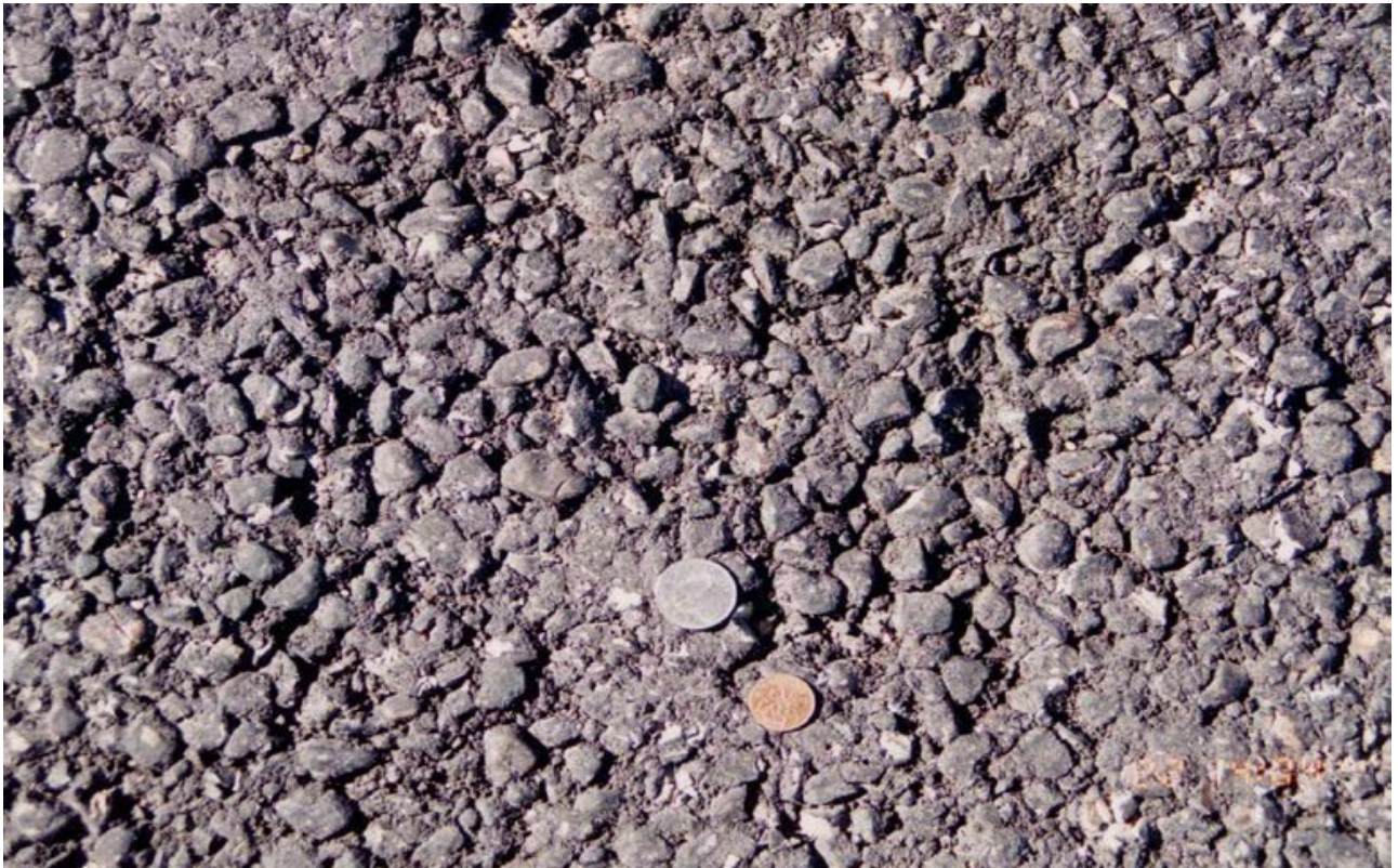
Figure 12 - Severe Segregation
