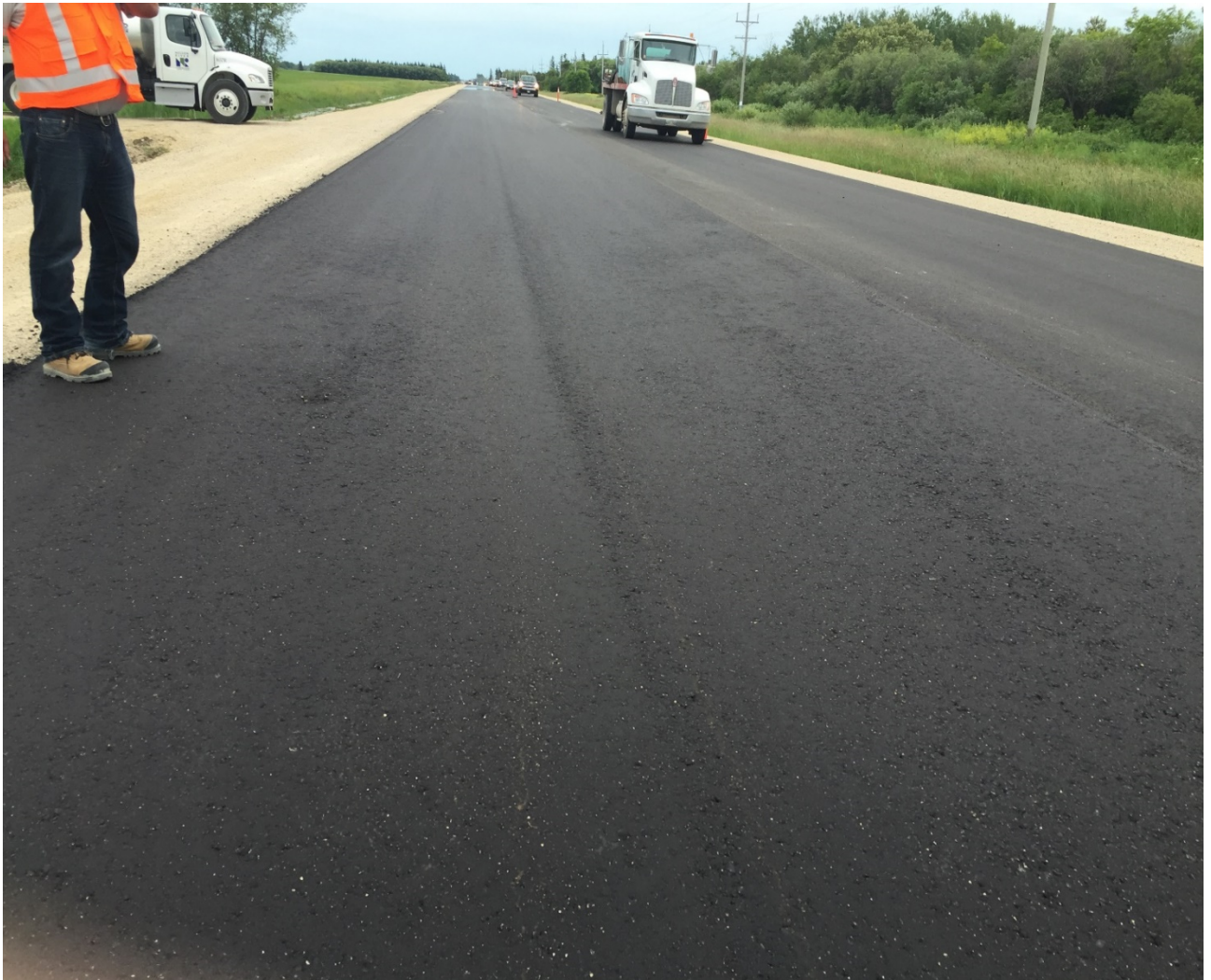
Figure 14 - Paver Streak
