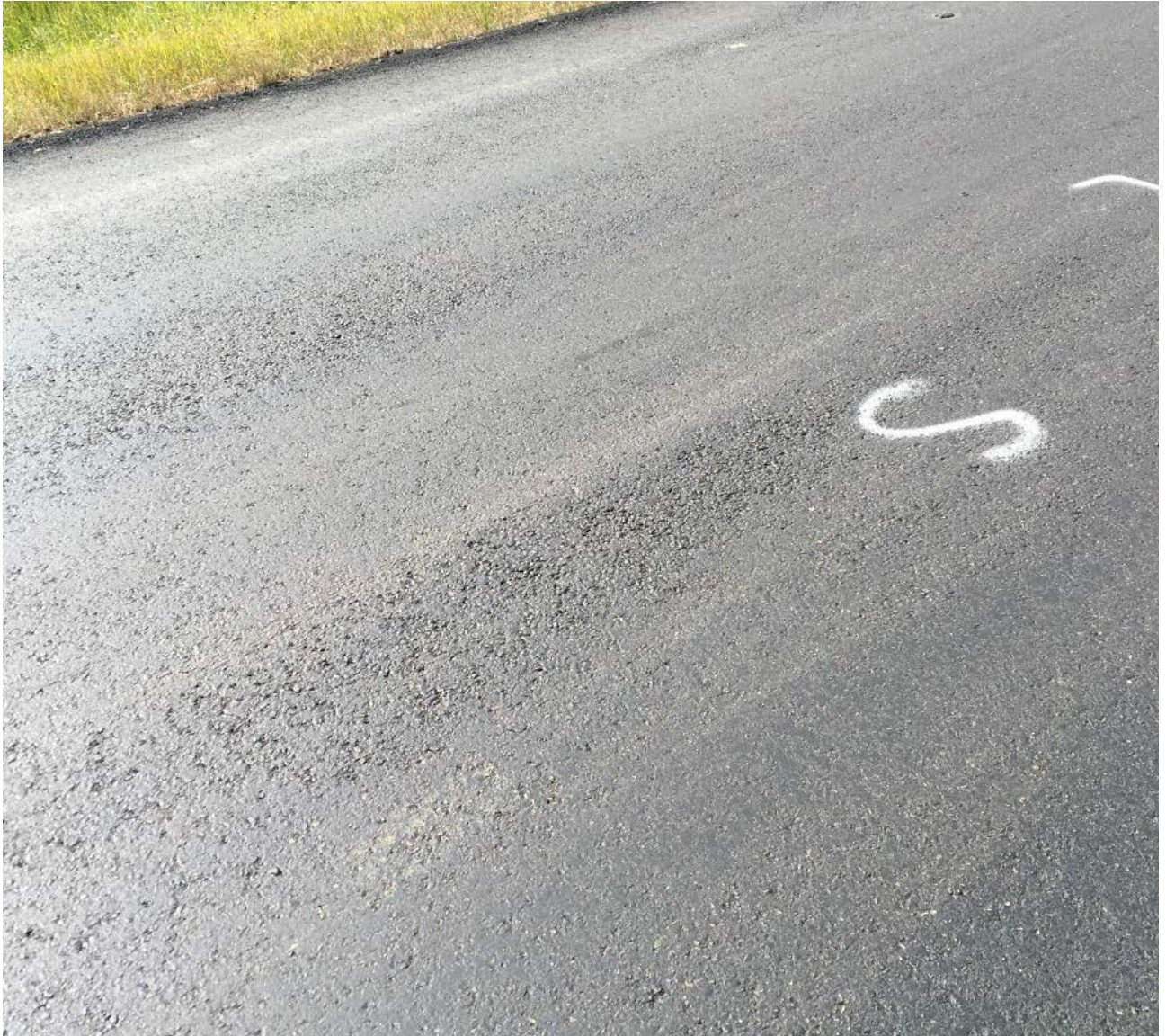
Figure 1- Slight Segregation
