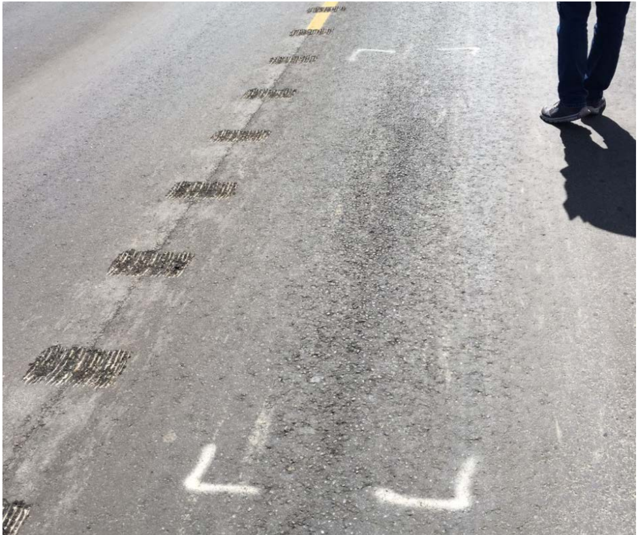
Figure 6 - Moderate Segregation
