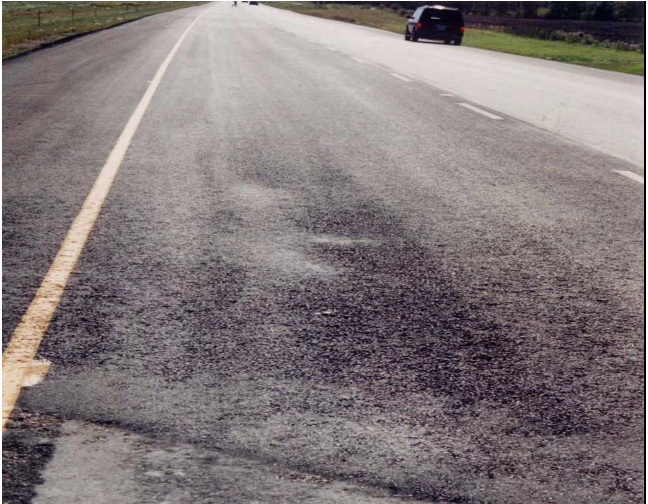
Figure 10 - Severe Segregation
