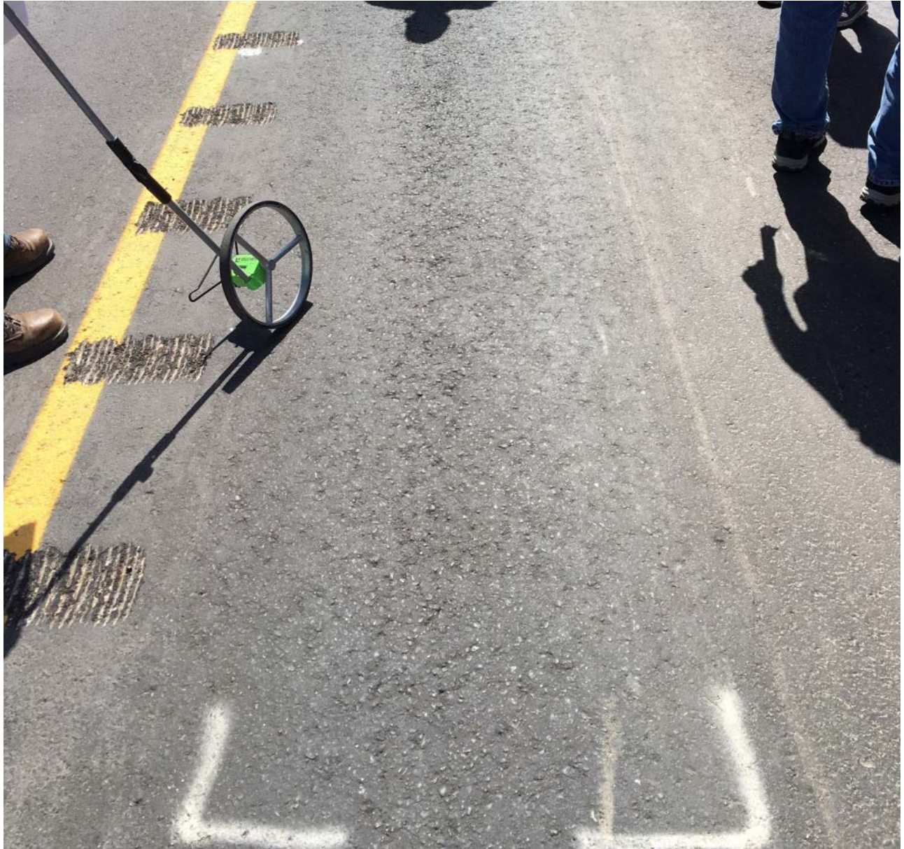
Figure 5 - Moderate Segregation
