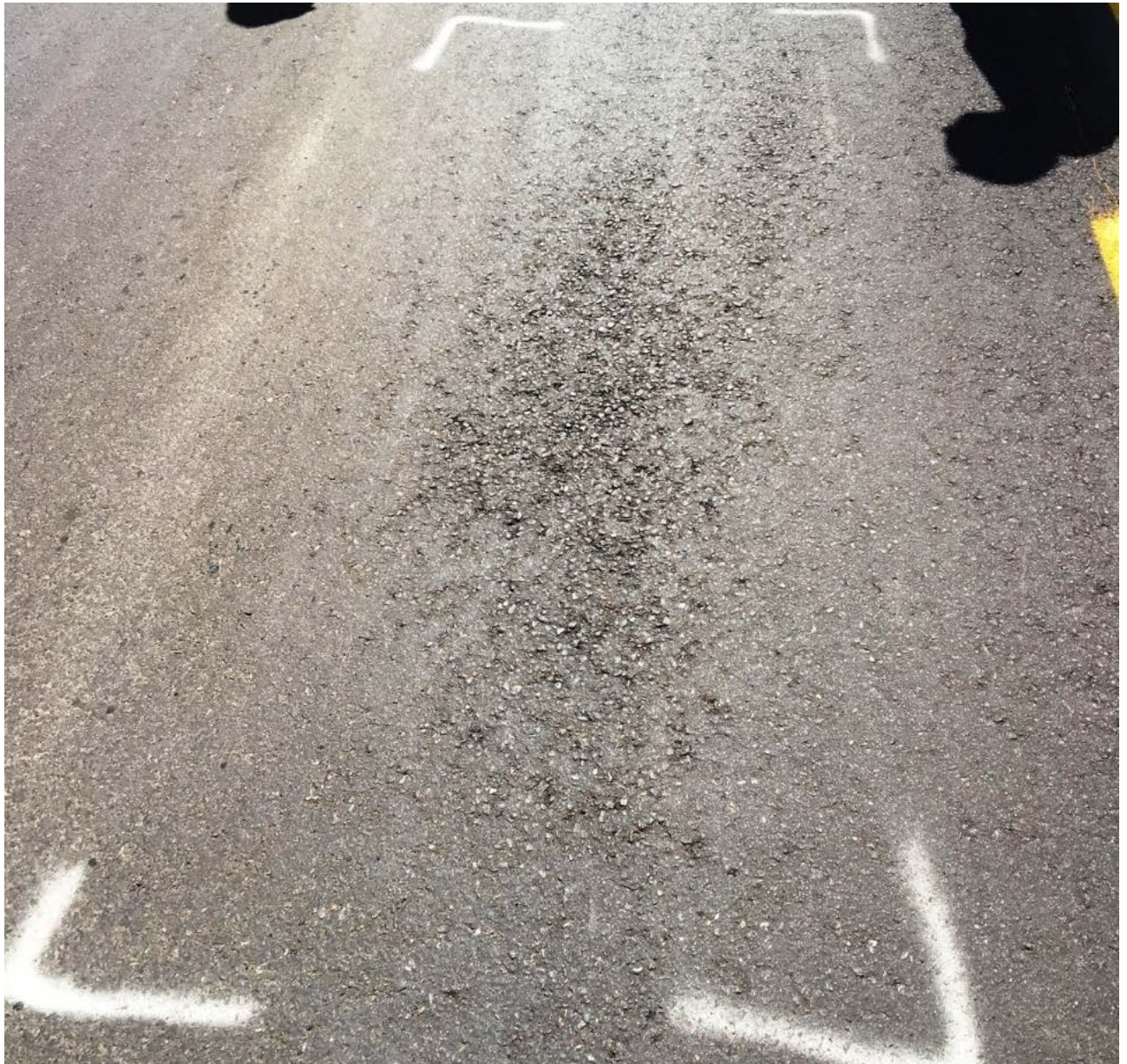
Figure 7 - Moderate Segregation
