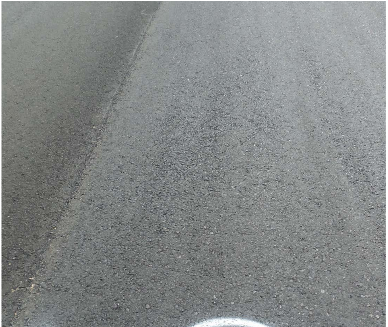
Figure 3 - Slight Segregation
