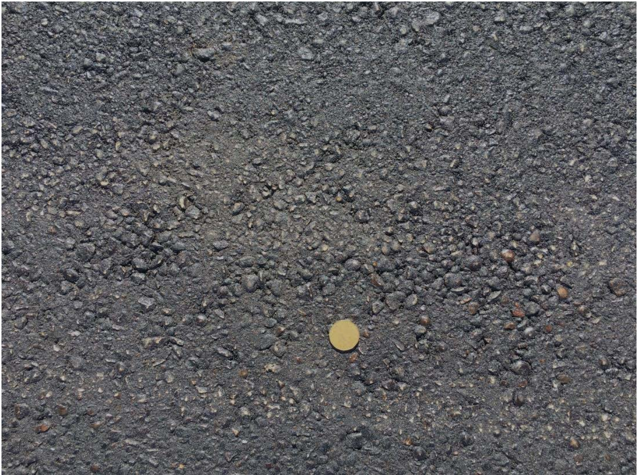
Figure 4 - Slight Segregation
