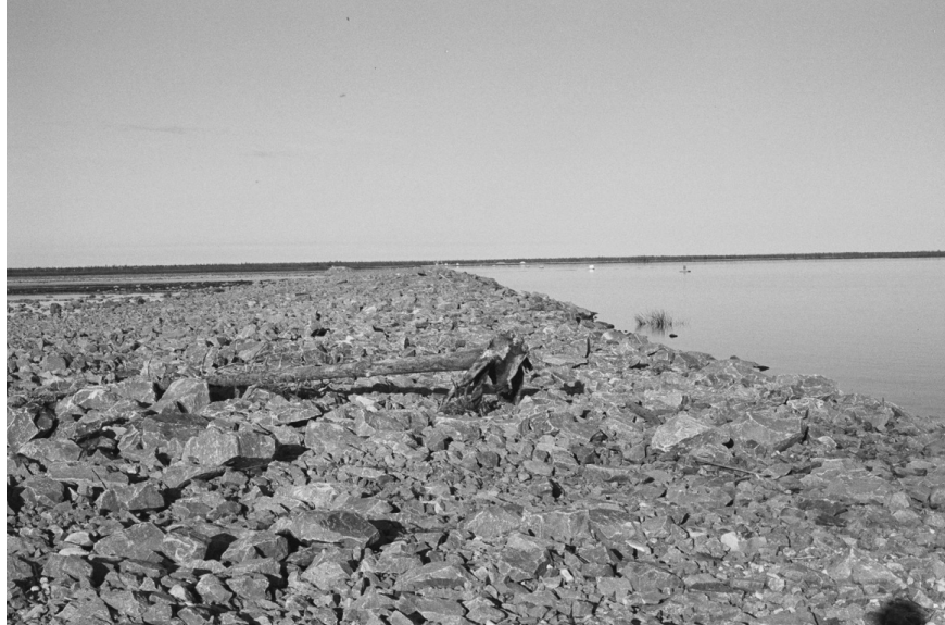
Figure GS-22-2: Churchill Weir constructed with Churchill Quartzite aggregate.
