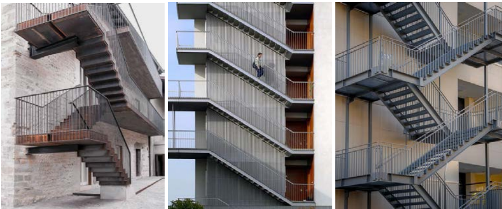
Figure 1: Open-air external metal staircase – Not allowed.
