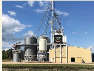
THE HEMP SENSE INC. FACILITY IN GILBERT PLAINS, MANITOBA.
