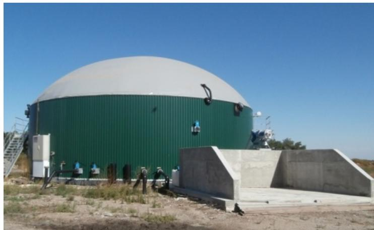
Figure 1. Anaerobic digester with solid digestate storage
