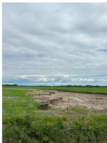
Flood Damage south of Minitonas, photo credit Nicole Clouson
