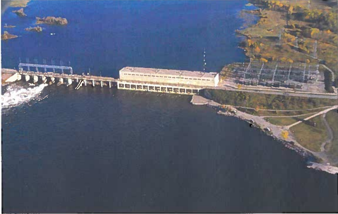
Photograph 1: Pine Falls Generating Station
