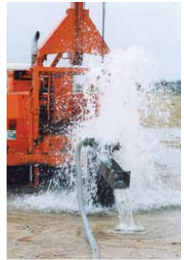
Developing a well by air lifting
