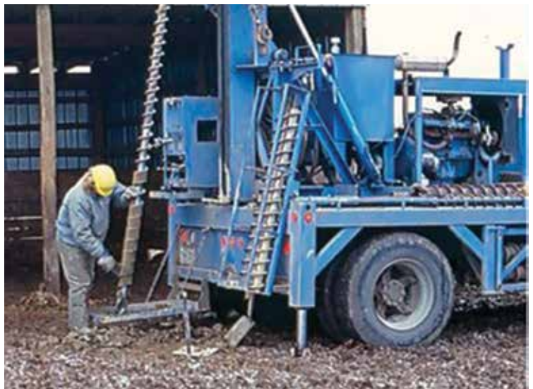
Drilling a test hole using an auger drill rig
