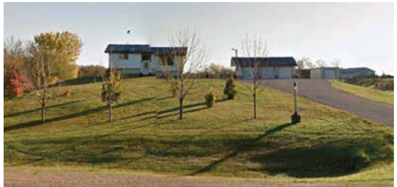
Well located on a pad above the flood protection level (Photo credit – Google Earth, October 2014)
