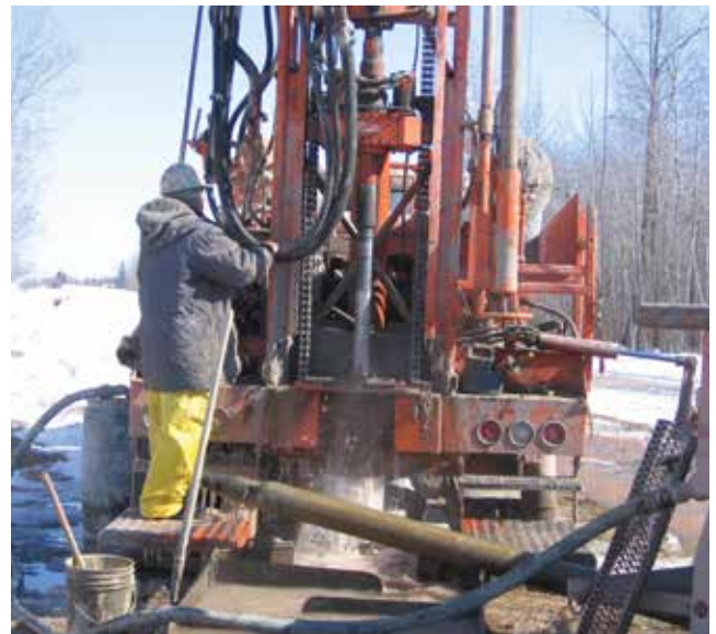
Drilling a provincial groundwater monitoring well
