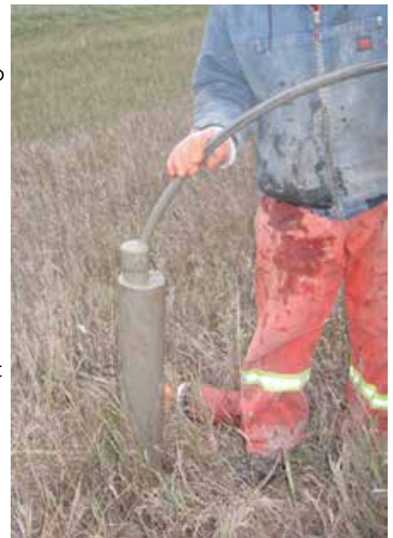
Sealing a small-diameter well using slurry grout
