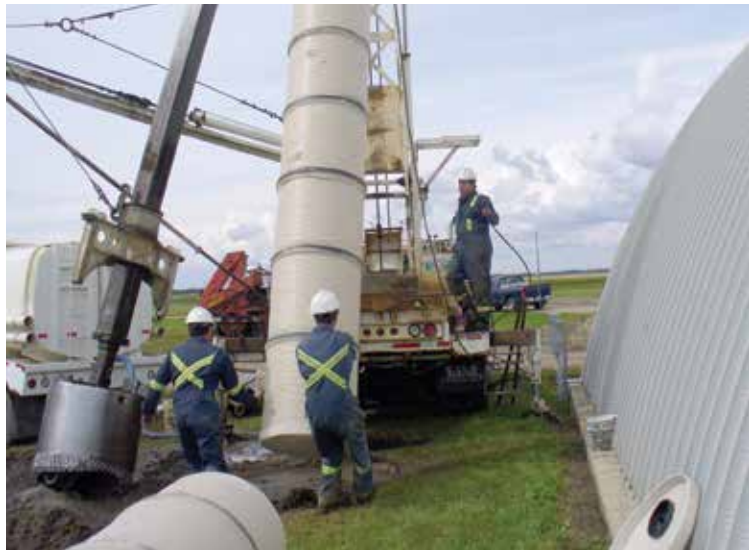
Constructing a large diameter production well
