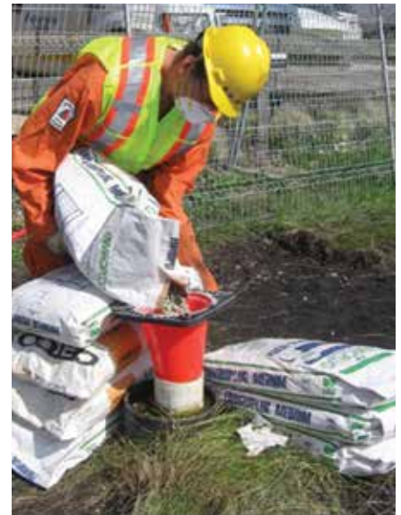
Sealing an abandoned water well
