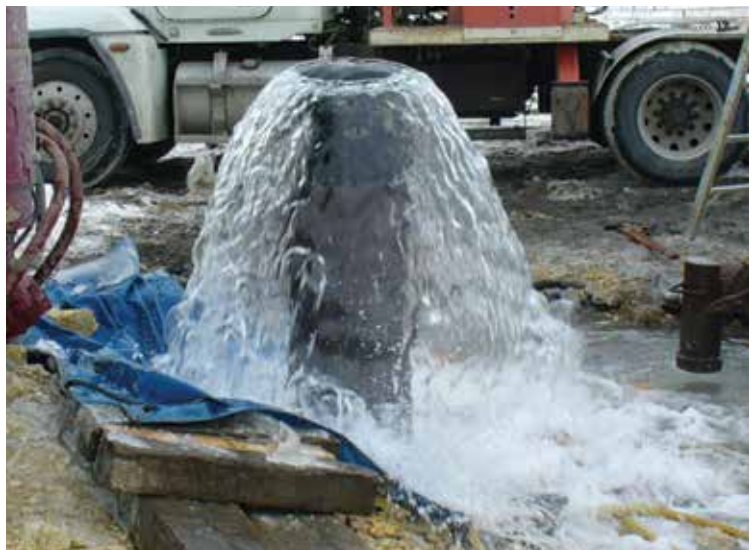
Constructing a flowing artesian well
