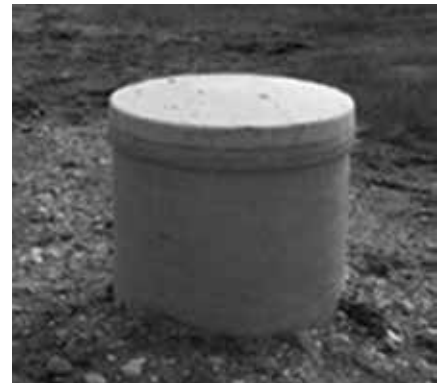
Well lid on a bored well (Photo Credit: Manitoba Water Well Association)
