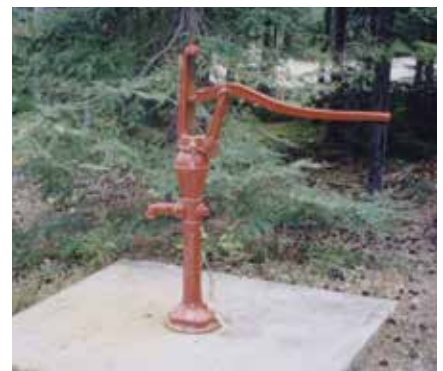
Hand pump with a concrete splash pad
