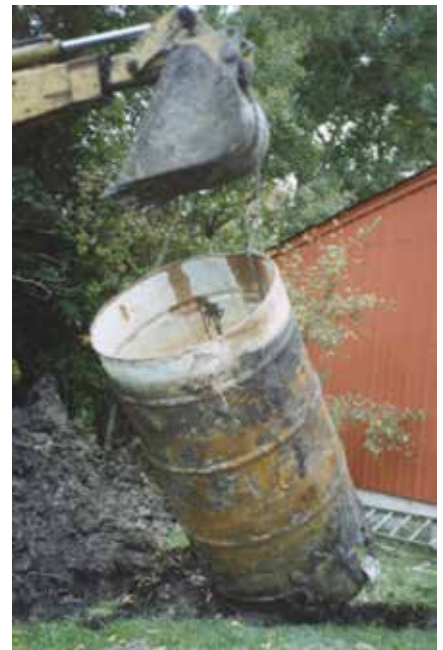
Removing a well pit cribbing
