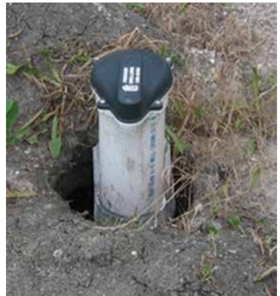
Open annular space outside a well casing
