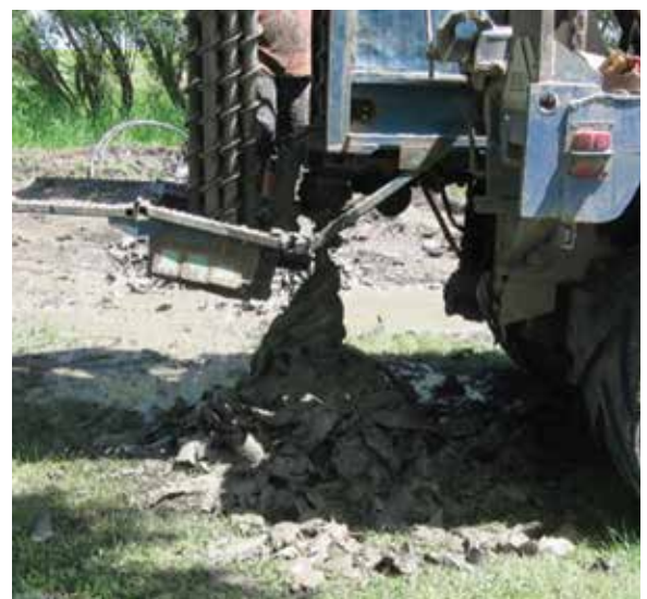
Drilling an auger hole for a closed loop geothermal system
