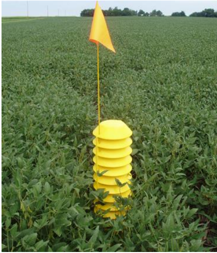
Figure 7: Tile riser in the field, left (Morrison, 2012), and construction of a blind inlet, right (Smith, Delaying Drainage from Prairie Potholes Protects Water Quality , 2013).
