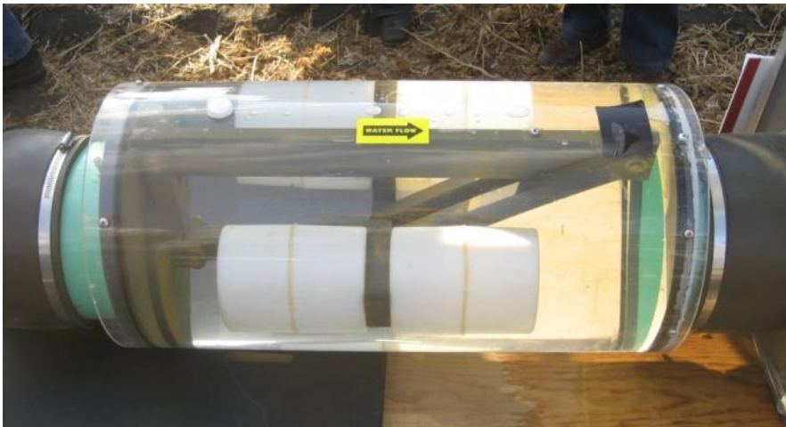
Figure 5: Water gate float-activated control valve (Cooley, 2011).
